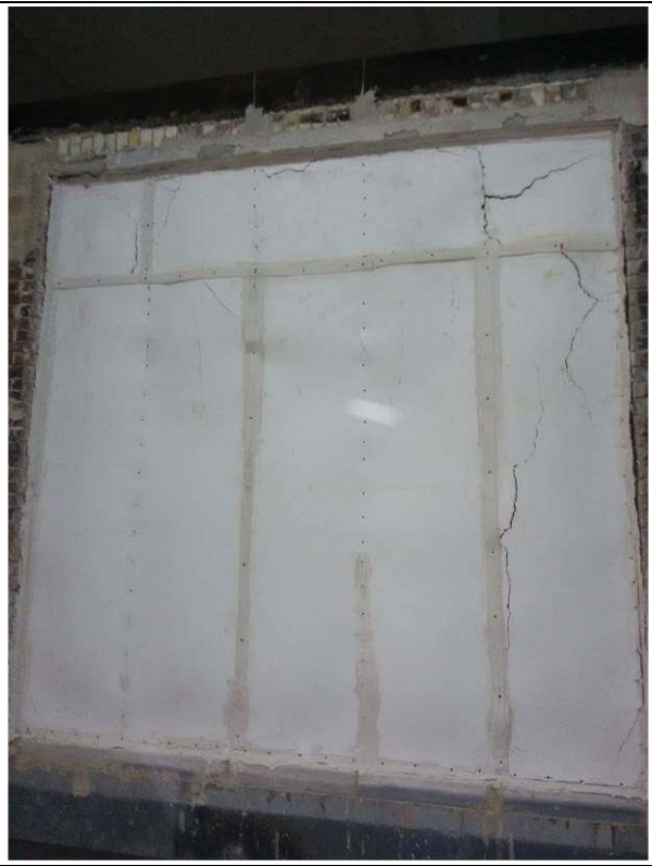
Exposed face after the test
